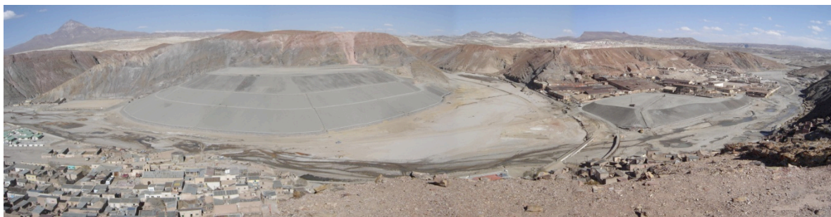
Figure 2. Panoramic view of the mitigation works carried out in Telamayú, 2004.
